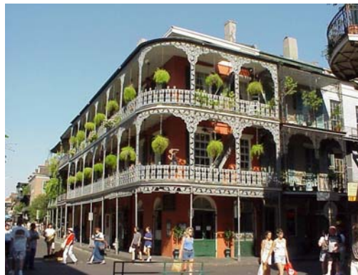
Old buildings—new buildings, we are your source for moisture problem resolution.
